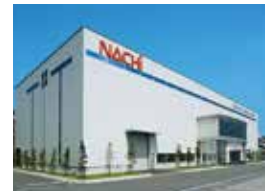
Special steel melting factory
