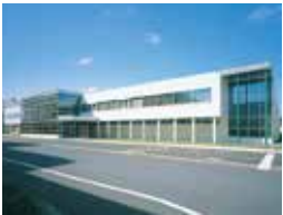
Internal broaches factory
