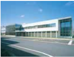
Internal broaches factory
