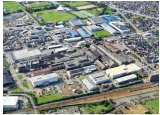
Products: Special Steels and Hydraulic Equipment Site Scale: 227,000m 2 Building: 126,000m 2
