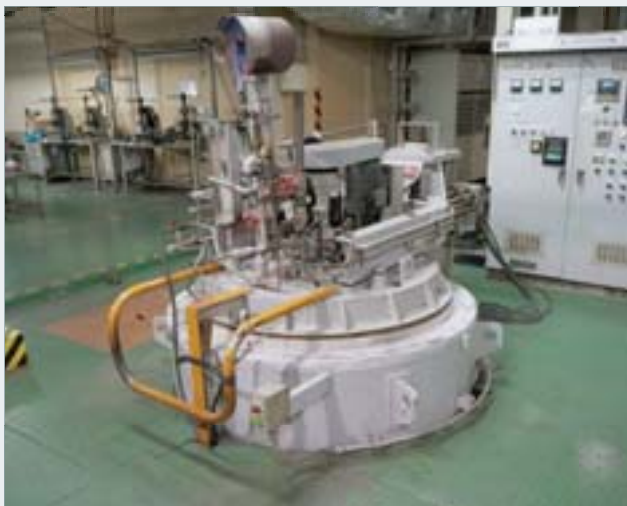
Pit type nitriding furnace
